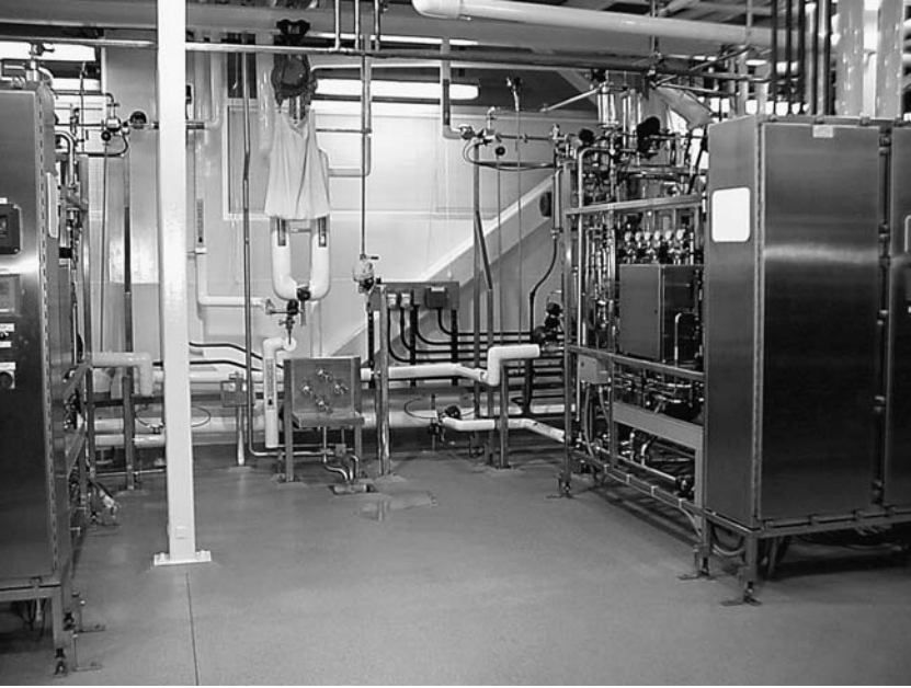
FIGURE 10 Photo of small transfer panel (such as TP-4) that supported pairs of bioreactors for the process of Figures 5 and 8.
