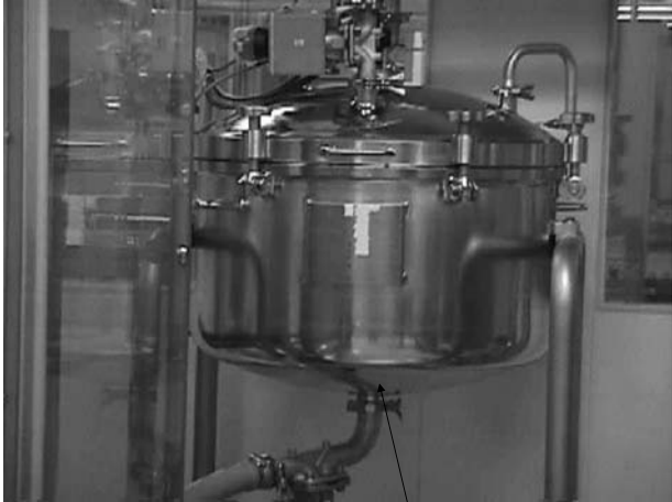
Filling Tank RT1
